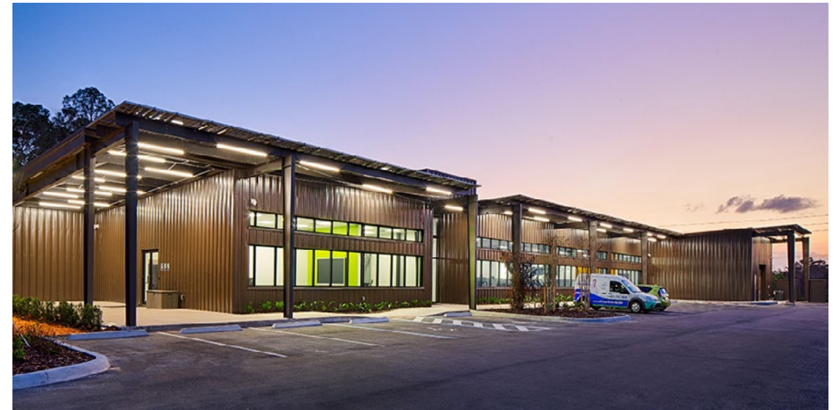
IMAGERY: Added canopy systems to add interest to basic PEMB construction.
