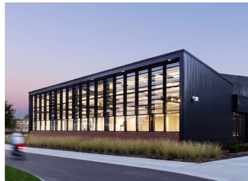
IMAGERY: Creating transparency within the solid PEMB forms adds interest and “lightness” to the simple metal boxes.
